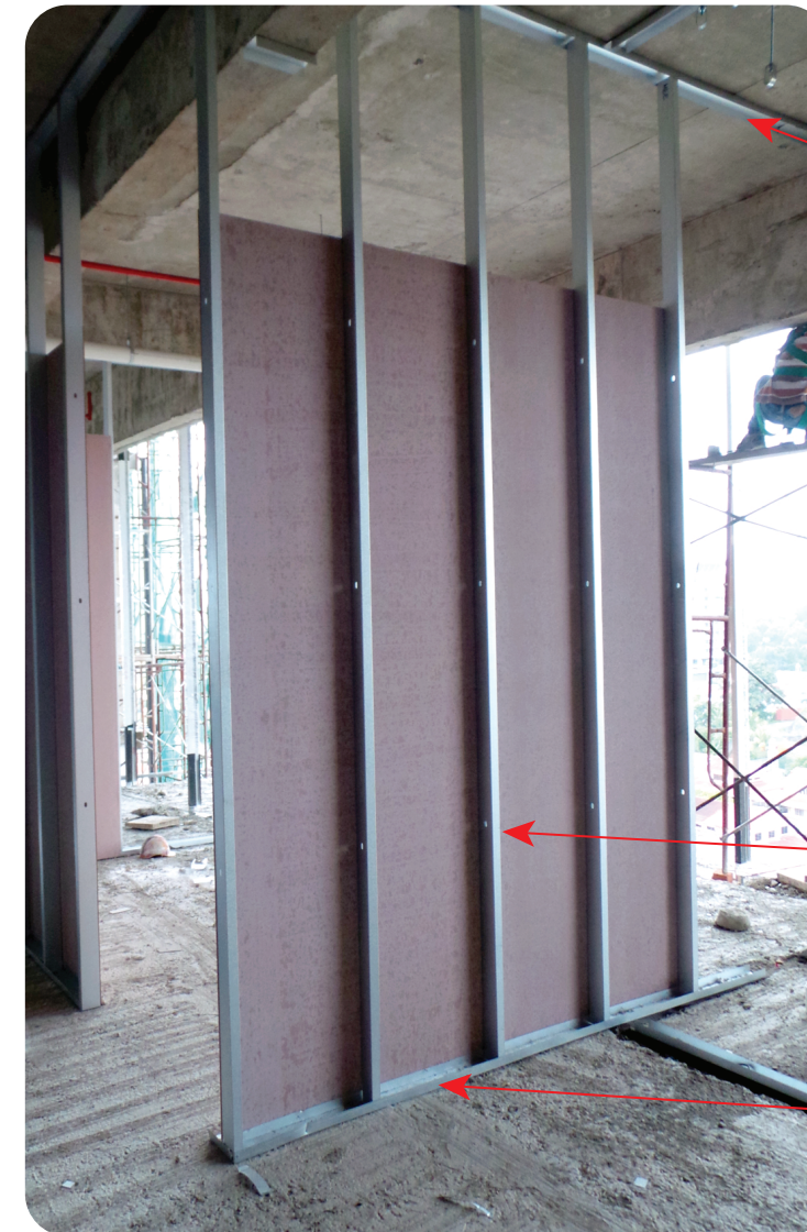
Photo shown C Stud, U Track & Top Head Track
