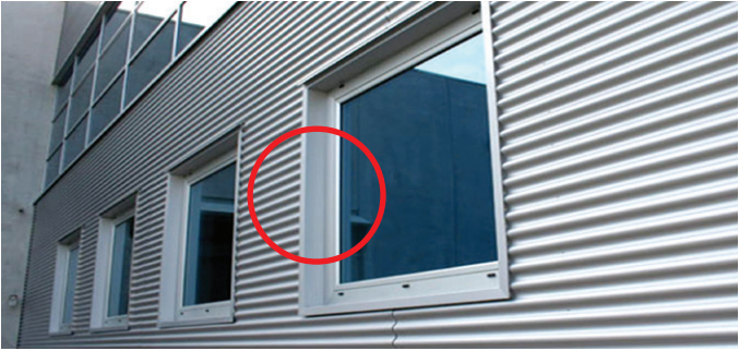
Window Frame Finishing
