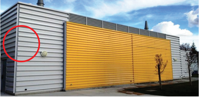
Workshop Cladding Finishing
