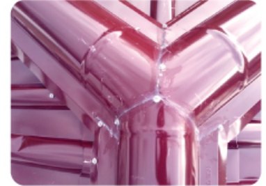
Figure 6 : Length Lapping Details
