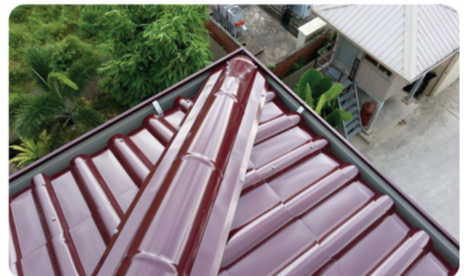
Besides using End Cap at the End of RRC 340, it also can do a bit of modification to slightly cover down the end.
